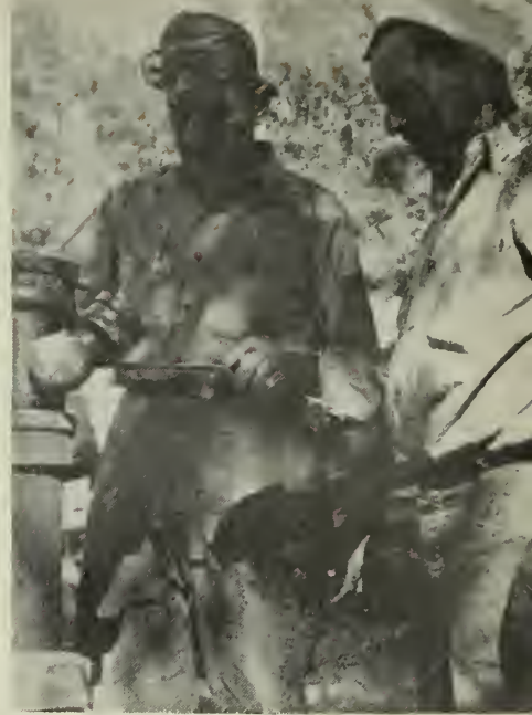
RESERVE Utilitymen get practical experience while building BSA camp.
